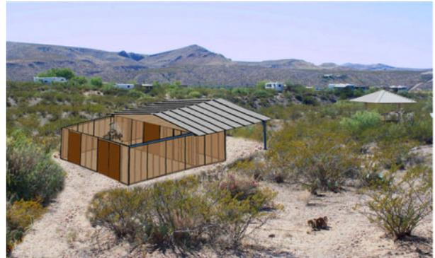
*The proposed design for ASLC's Observatory includes a 16 x 20 foot roll-off roof and a 6 x 14 foot warm room.*
